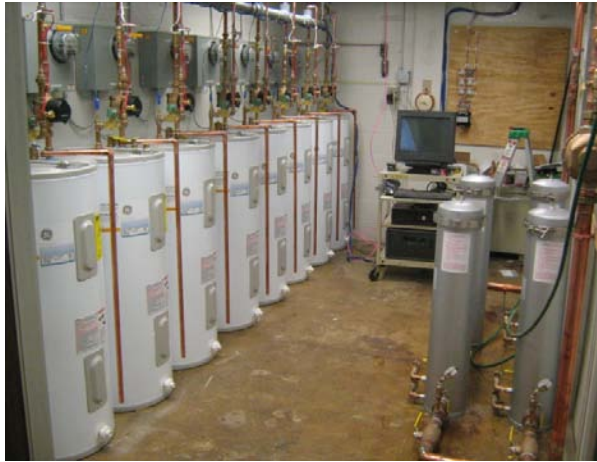
Figure 4-3. Electric Water Heaters
